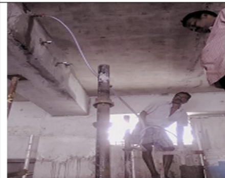
INJECTION GROUTING
